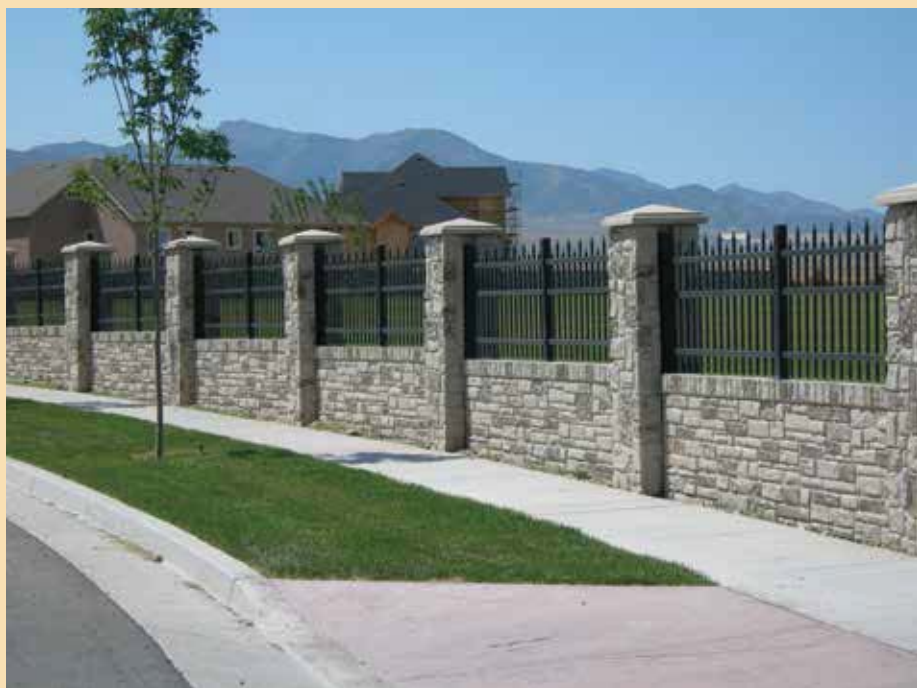
TOP: ASHLAR BOTTOM: ASHLAR COLUMNS WITH LEDGE STONE/WROUGHT IRON PANELS
